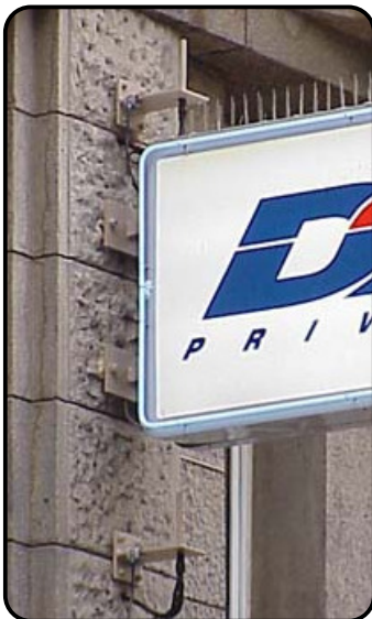
Very hard to find: A micro cell on a building wall, above and below a billboard
