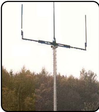
Omnidirectional base station with a single cell
